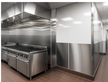
Quarry tile with coved base, stainless and FRP wall panels, washable ceiling grid.
