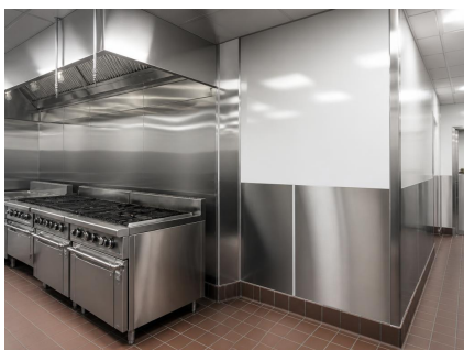
Quarry tile with coved base, stainless and FRP wall panels, washable ceiling grid.
