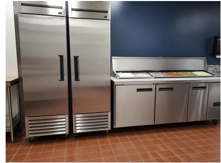
Reach-in cooler and freezer with undercounter prep rail.
