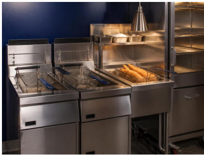
Fry line: twin-vat fryers, filter cart clearance, dump and crisping station.
